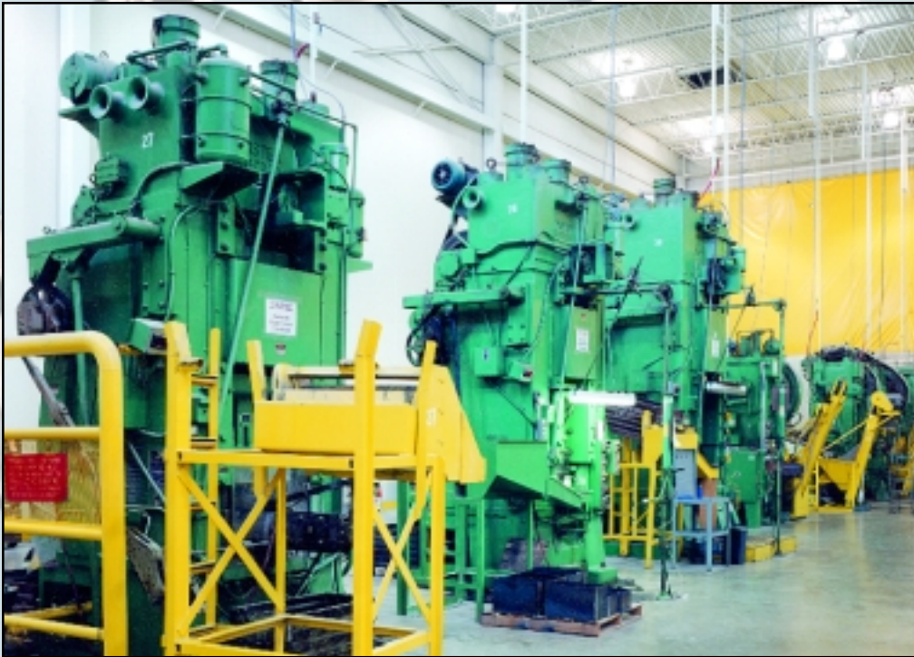
Metal Forming and Coining utilizes several Minster knuckle joint presses in its cold forming operations.
