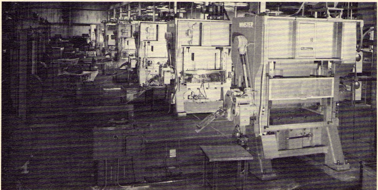
Lamination press line at A. O. Smith. Press in foreground is in process of installation.
