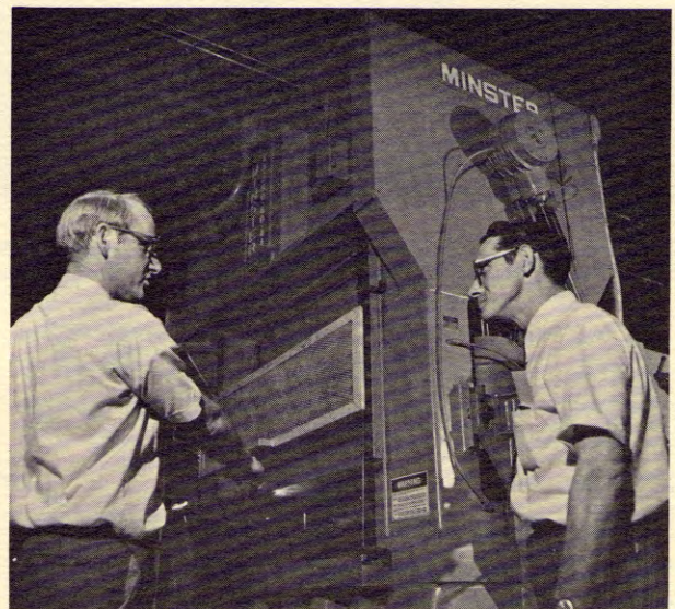
Norm Maggard, Manufacturing Engineer, left, and Al Tufono, Maintenance Superintendent, check press installation progress.
